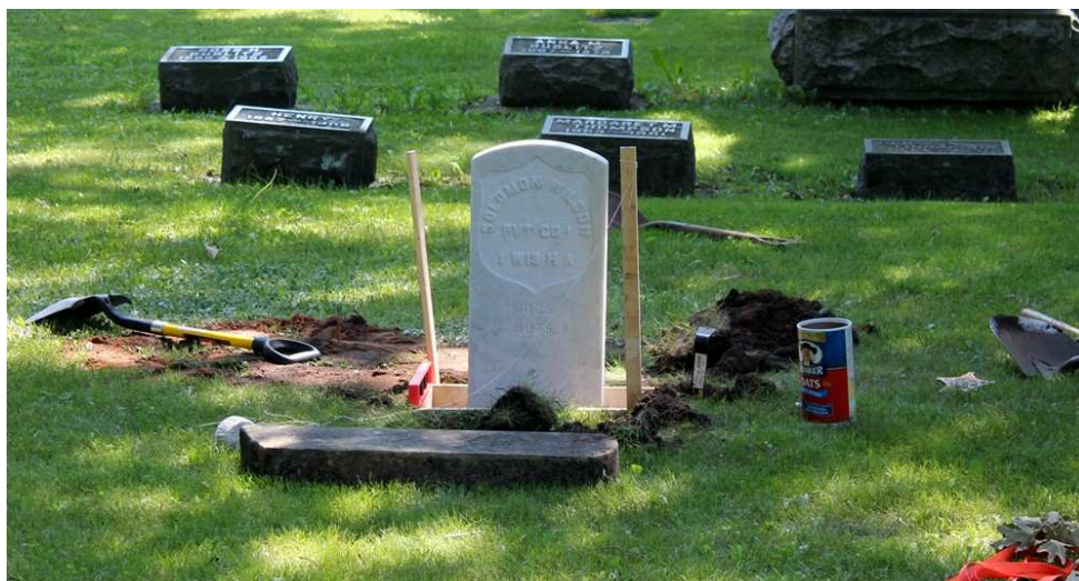
The first stone is leveled and the next step is to mix & pour the cement.
